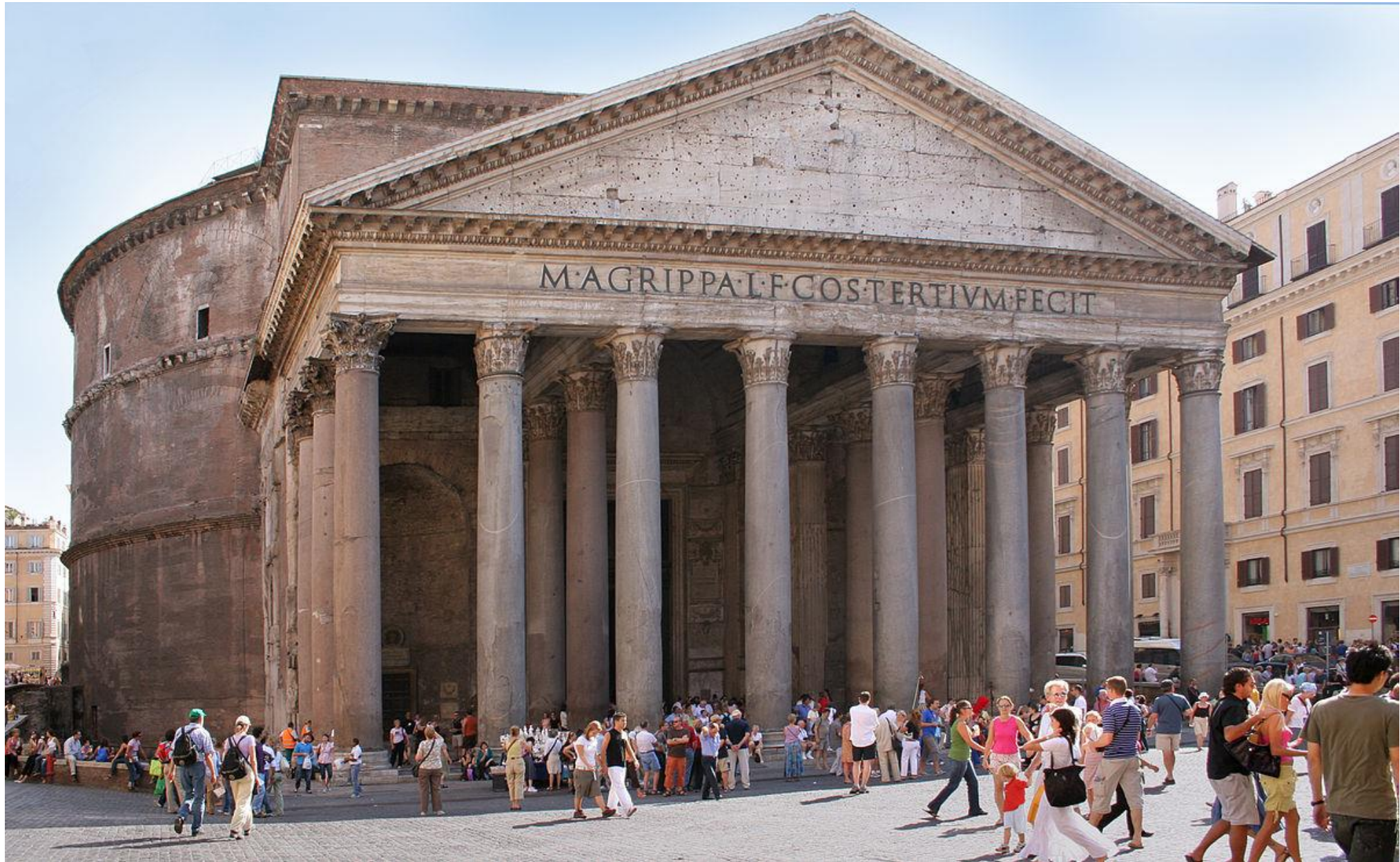
The Pantheon C.130, travertine, brick, lava-stone (tufa), pumice, marble, Rome
